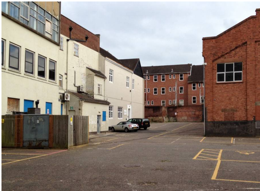
Photograph A – View of Electric Substation "Duke Street No 1"
