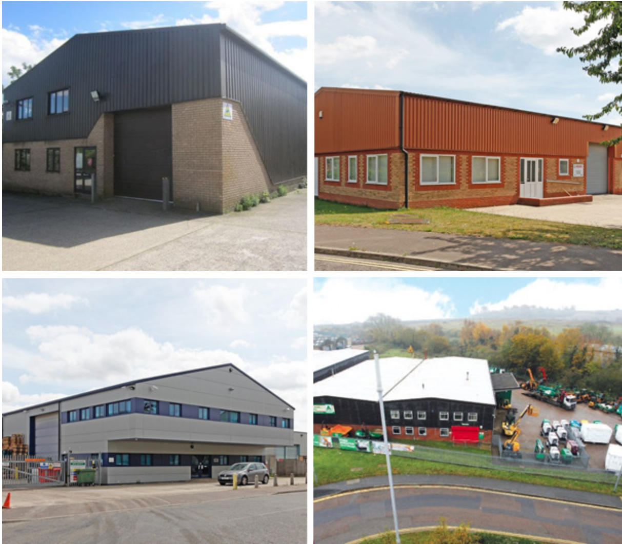
Figure 16: Industrial Units in Greater Norwich
