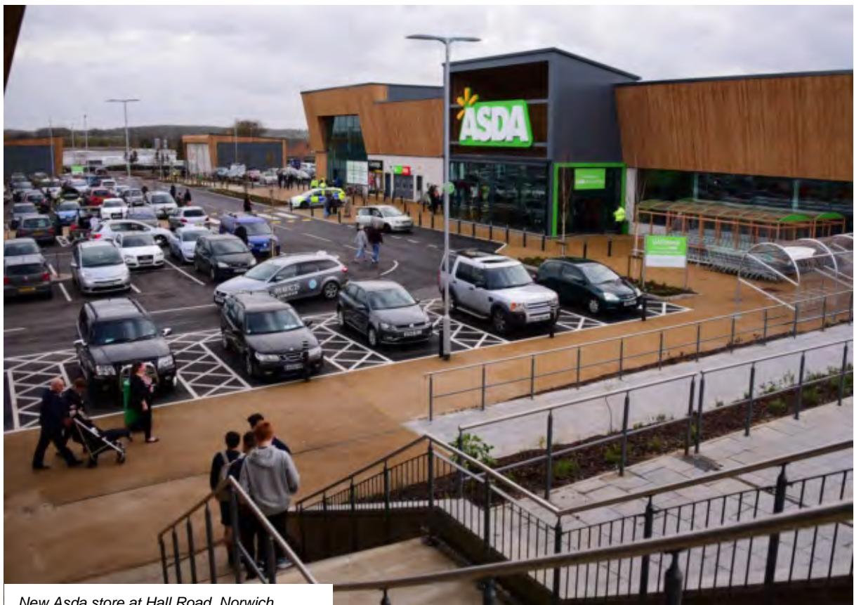
New Asda store at Hall Road, Norwich
