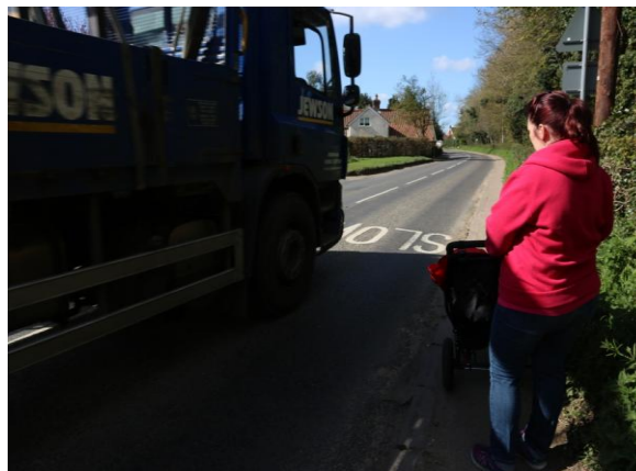
Photograph: Narrow footpath along the B1113 (65cm) and with no kerb
