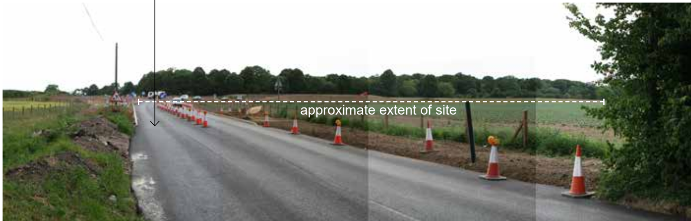
Figure 36 Viewpoint 14. Looking south-west on Salhouse Road, approximately 1km from the site. Earthworks for the Northern Distributor Road are seen in the near distance. The site is completely obscured by intervening vegetation.
