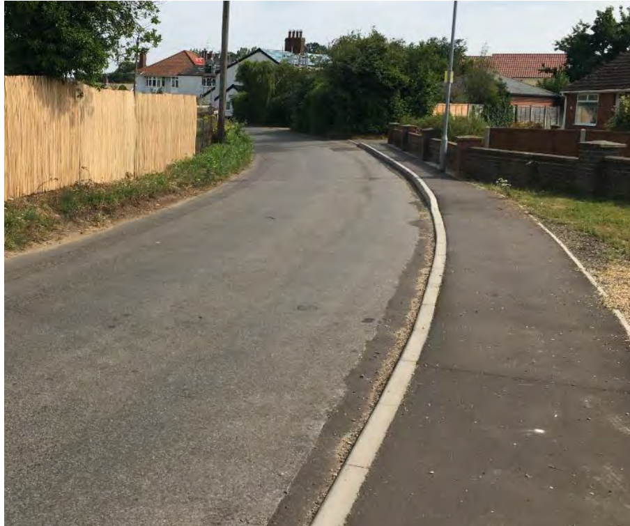
Photo 1 – Existing Footway on Hardingham Road.
