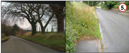
BURGH ROAD FOOTWAY: NEW SECTION OF FOOTWAY TO BE PROVIDED ON THE NORTH SIDE OF THE CARRIAGEWAY ALLOWING A CONTINUOUS PEDESTRIAN LINK TO/FROM THE TOWN CENTRE
