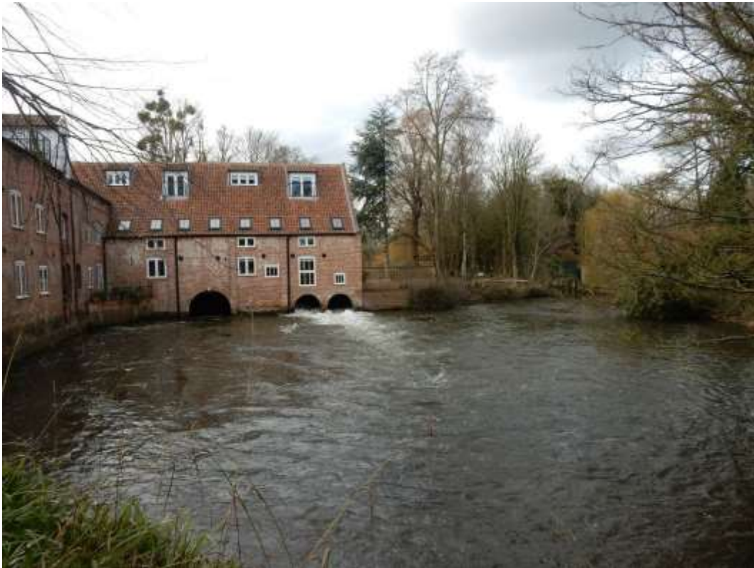
Plate 5: Former watermill and mill pond, looking west
