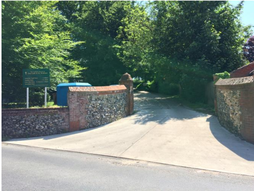
Figure 23: A view of the entrance gate to the church of Our Lady and Saint Walstan from Town House Road. A number of large trees screen the church and hence it is not visible from the road.
