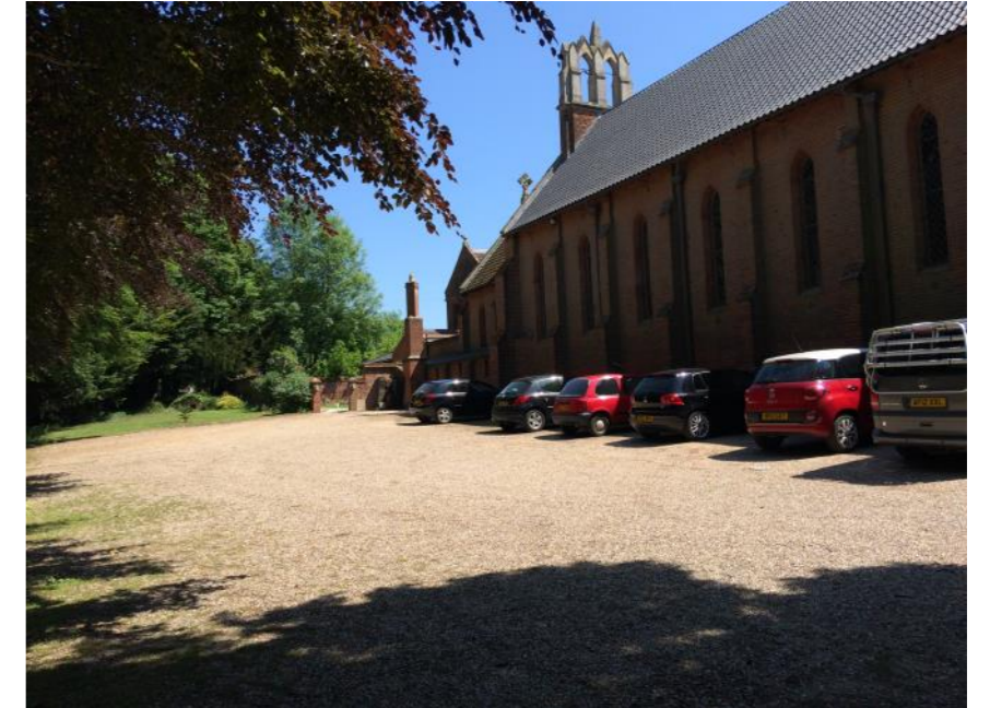
Figure 25: A view of the car parking area which is also located in the northern section of the churchyard.
