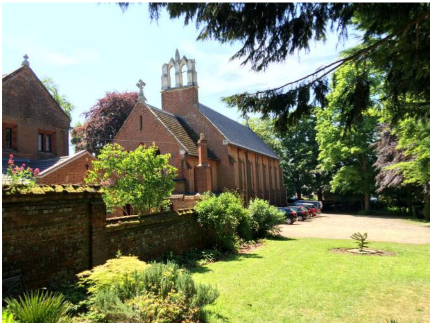
Figure 26: A view of the church's east end from the northeast.
