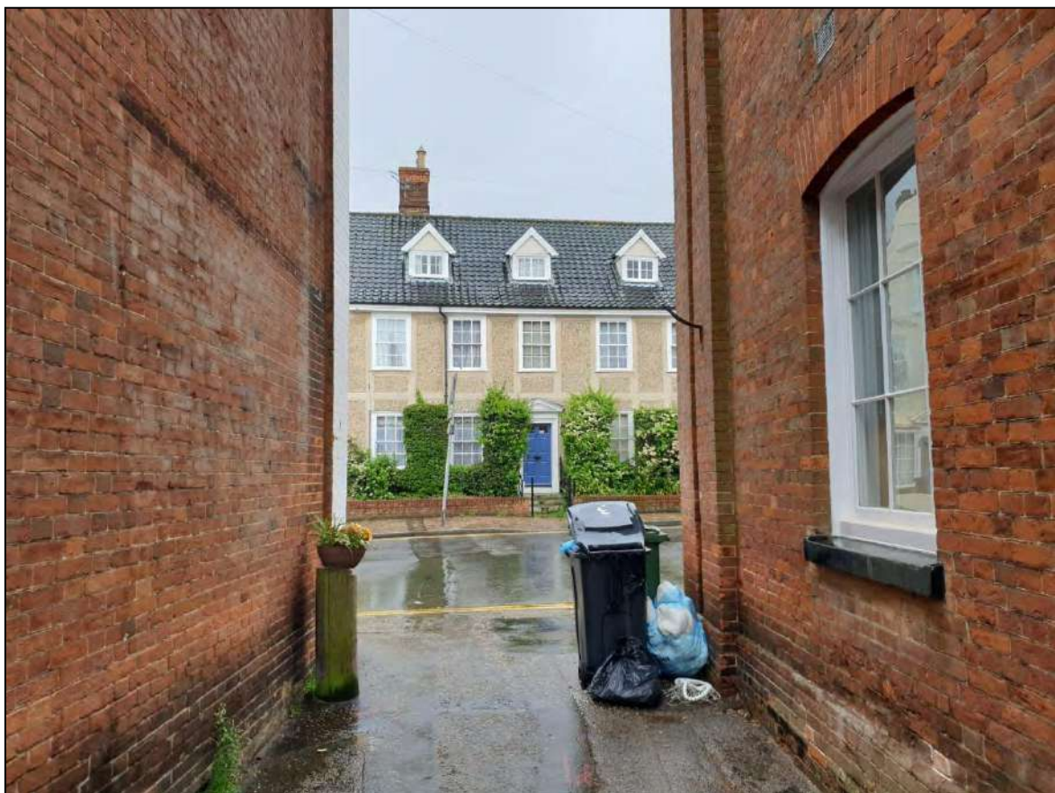
DP 38. View across Old Market Place from Green Dragon Lane with the Grade II listed Post Office on the right of the image and the Grade II listed 3 & 5 Old Market Place on the left of the image
