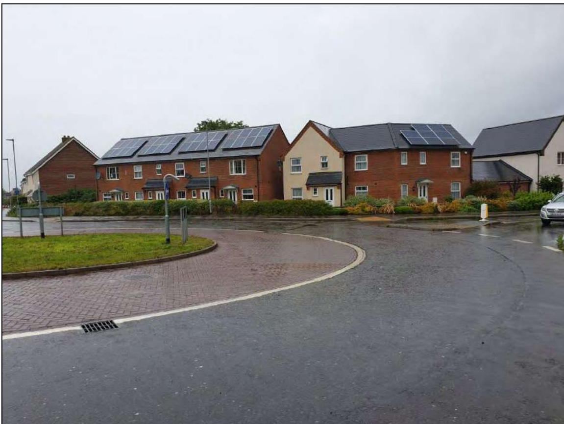
DP 4. View north-west towards Harleston town centre from the same location as DP 3
