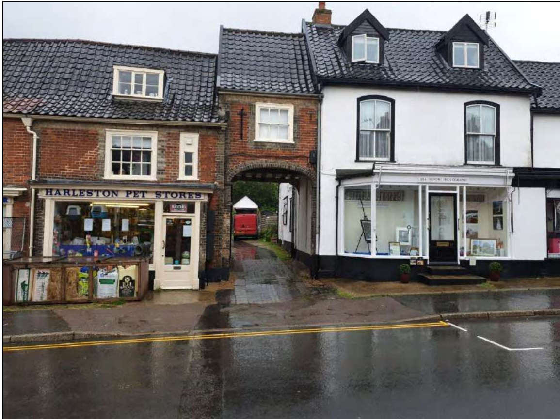
DP 39. View towards the proposed development site incorporating No. 14 and Nos. 16 & 18 Old Market Place
