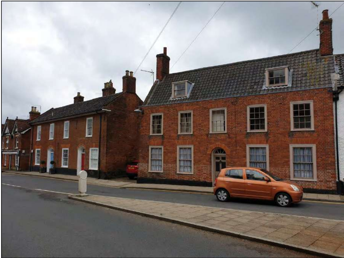
DP 27. View towards the proposed development site from the junction of The Thoroughfare and Broad Street, incorporating heritage assets in this area.
