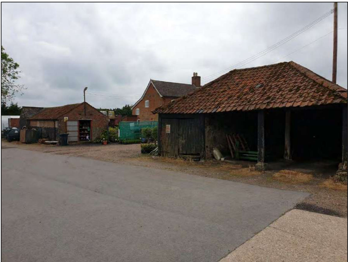
DP8. View south-east of farm buildings located within the centre of the proposed development site
