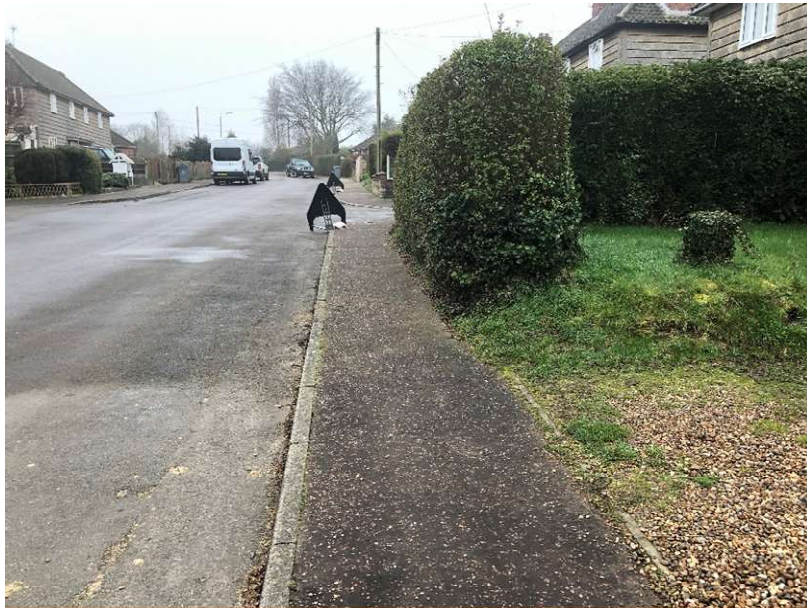
Figure 5-2 Le Neve Road – Northbound View
