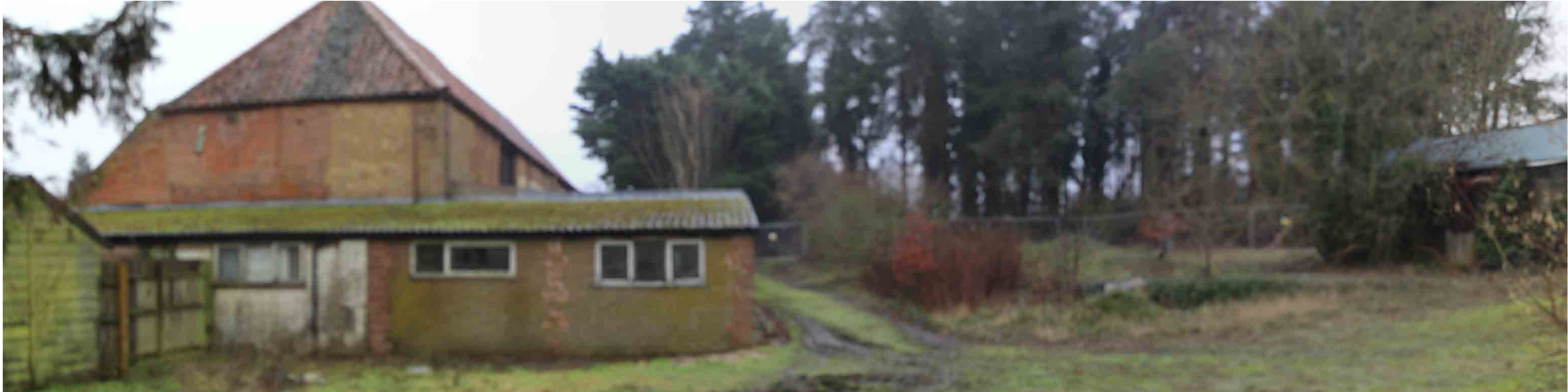
Photo Viewpoint D: Northerly view within the site of the derelict farm buildings
