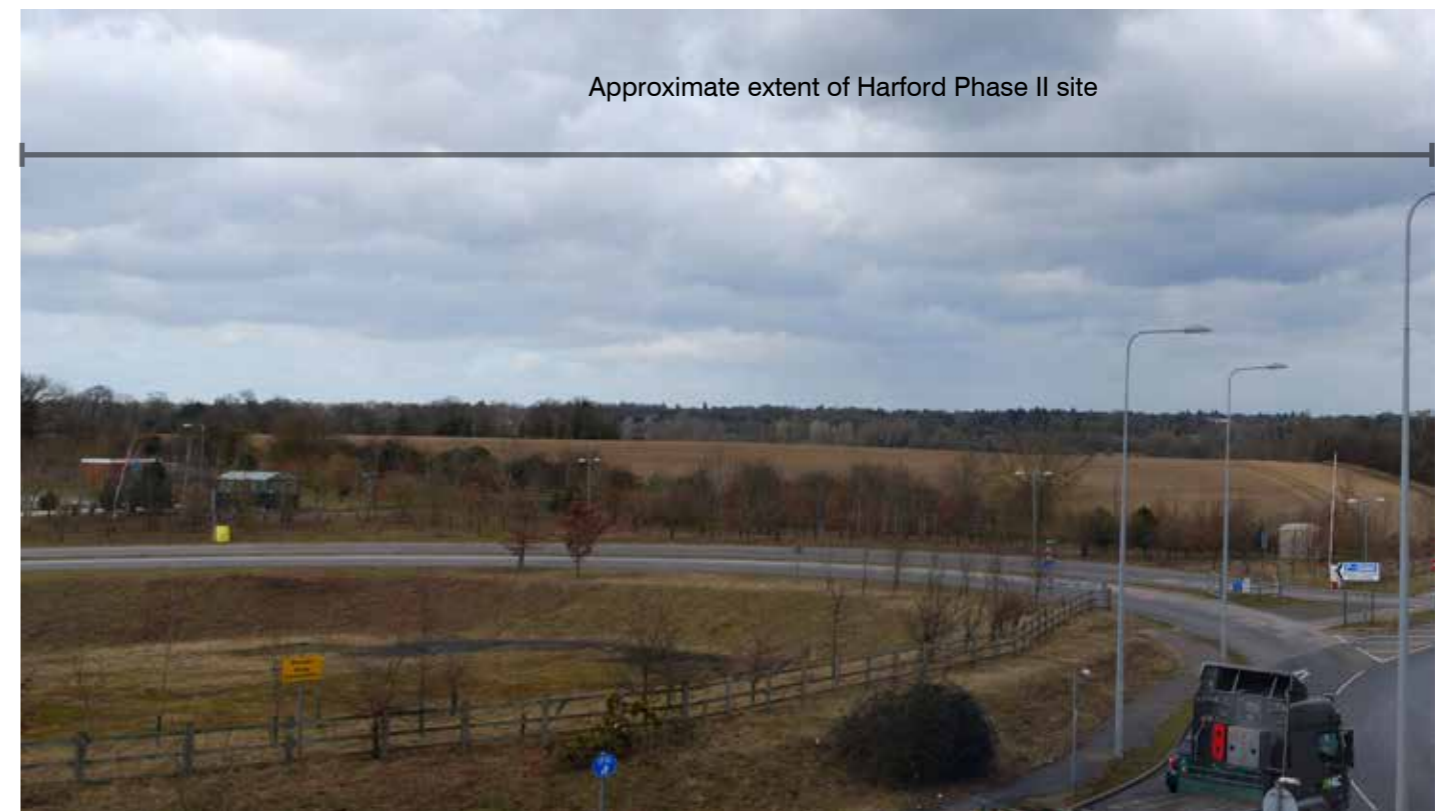
Viewpoint 4 - view taken from A47 Norwich Southern Bypass, above the junction with A140, looking north west towards the Site at approximately 130m distance. From this viewpoint the full extent of the new development will be visible.
