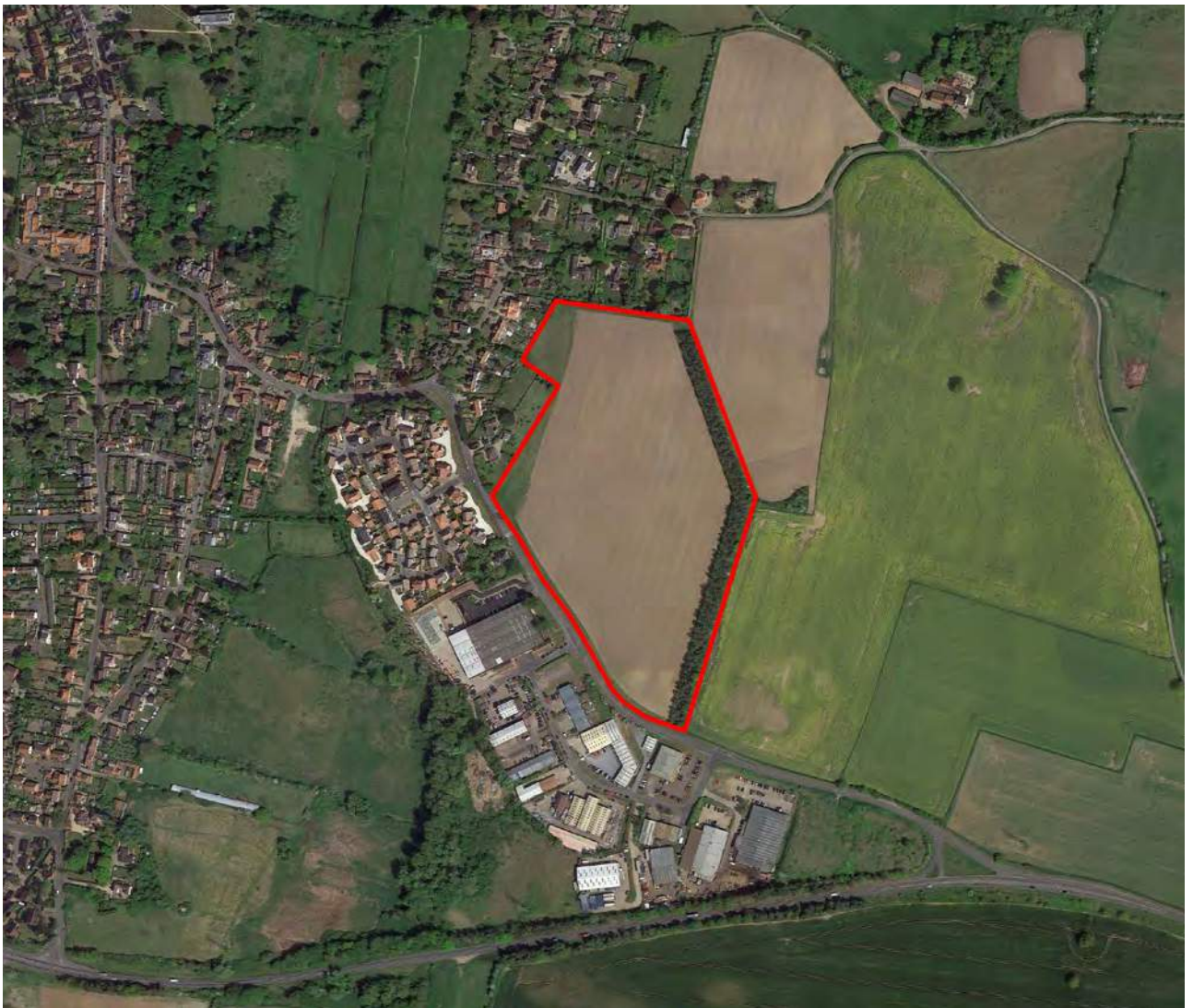
Aerial view of the application site
